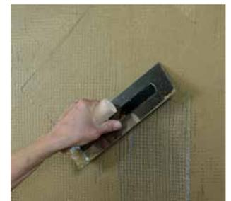
Drywall board made of clay and hemp for planking wood and metal elements within interior walls, skirting, ceiling and roof surfaces. CLAYTEC Greentech 700 is solid and stable, sharp-edged and dimensionally accurate. It has the best constructional biological properties. The drywall substructure grid is 62.5 cm. Its resistance to water also allows applications of thick clay plaster layers.
