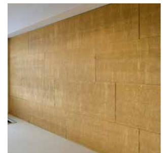
Drywall clayboards for planking wood and metal post and beam constructions within interior walls, facing, ceiling and roof surfaces. The CLAYTEC clayboard is a drywall board and a clay plaster in one. It was developed based on practical building experience and has been available on the market for 20 years. With a density of 700 kg/m<sup>3</sup> it provides a clay mass which is easy to handle.
